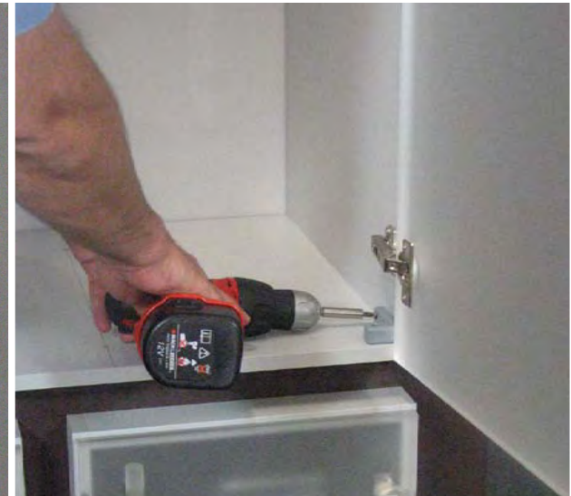
2. Screw on pull-out profile
