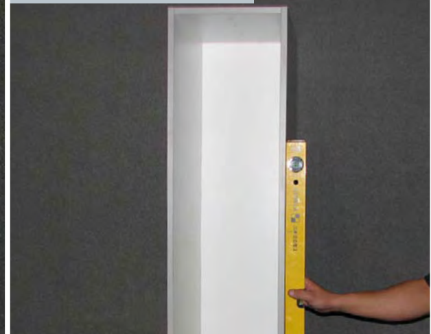
2. Align unit using spirit level
